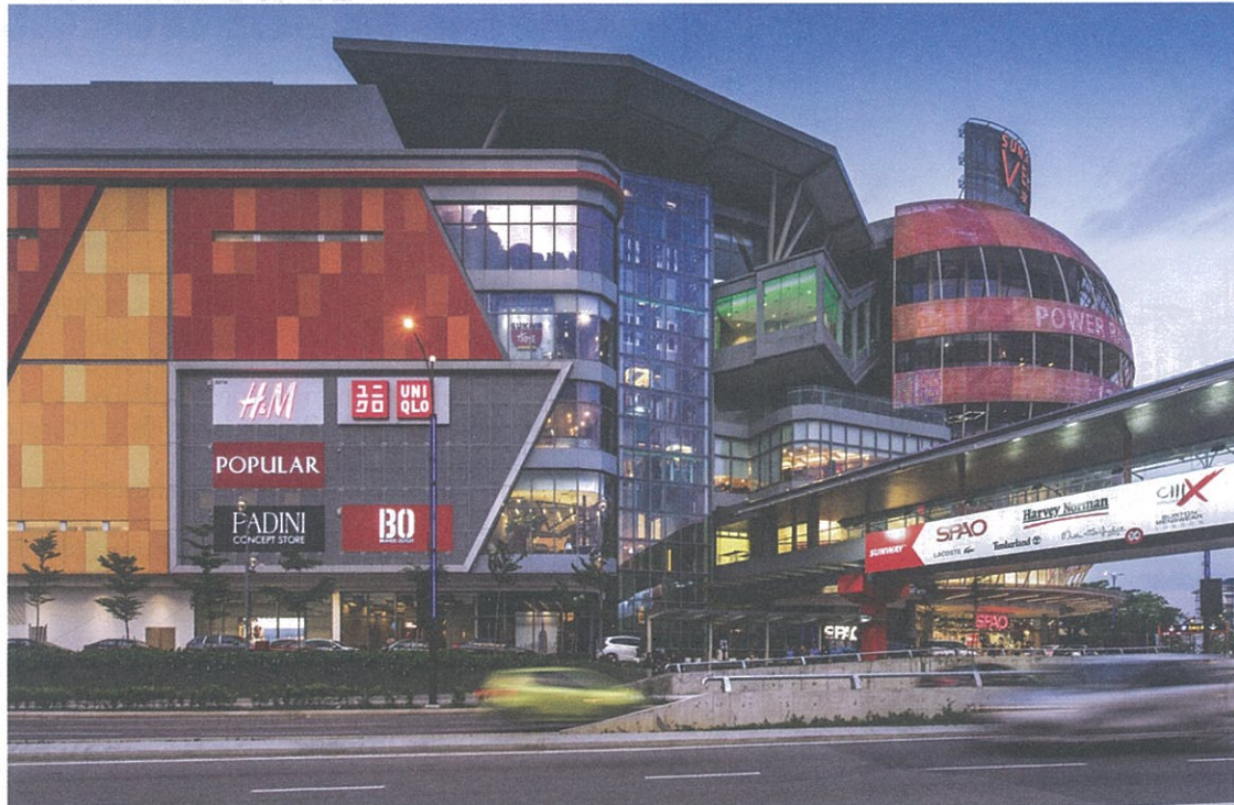
Sunway Velocity has an inviting and exciting frontage design that serves to draw shoppers
