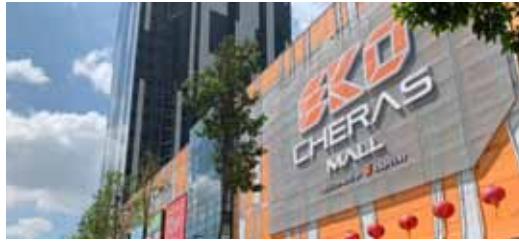
EkoCheras Mall's exterior facade
