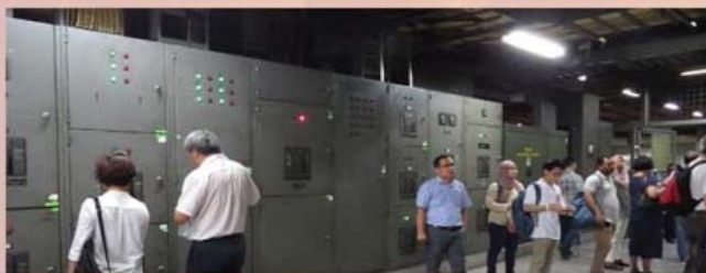
Checking out the M&E installations
